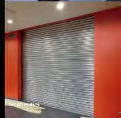
TM120 Fire shutter with 50 mm flat lath option
