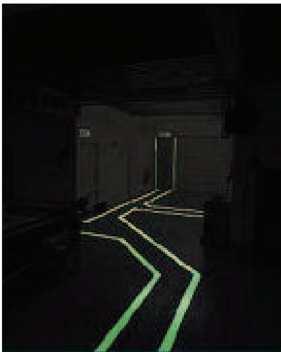
Figure 53: A 'way-guidance' system
