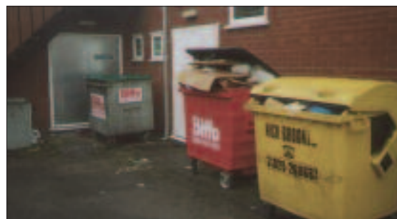
Figure 12: Bins next to a building (courtesy of Cheshire fire and rescue service)
