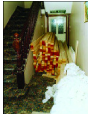
Figure 9: A blocked corridor with incorrect signage
