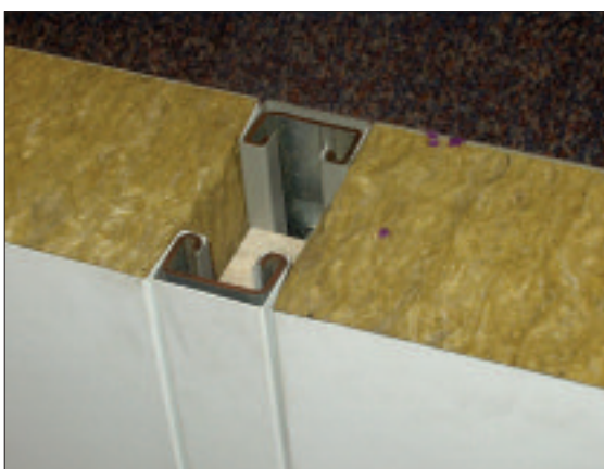
Figure 17: Insulated core panels – internal panel
